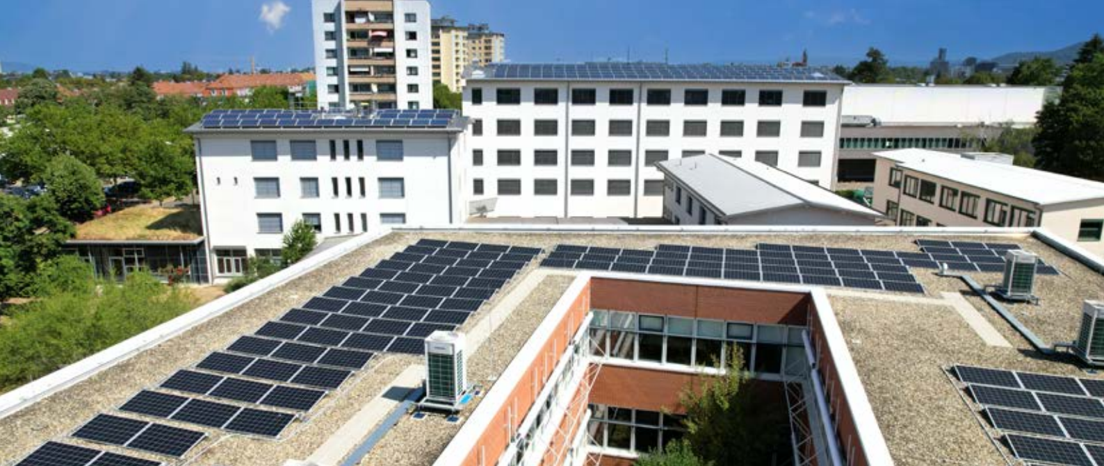
Figure 6: Photovoltaic systems installed on the roofs of our headquarters in Freiburg
