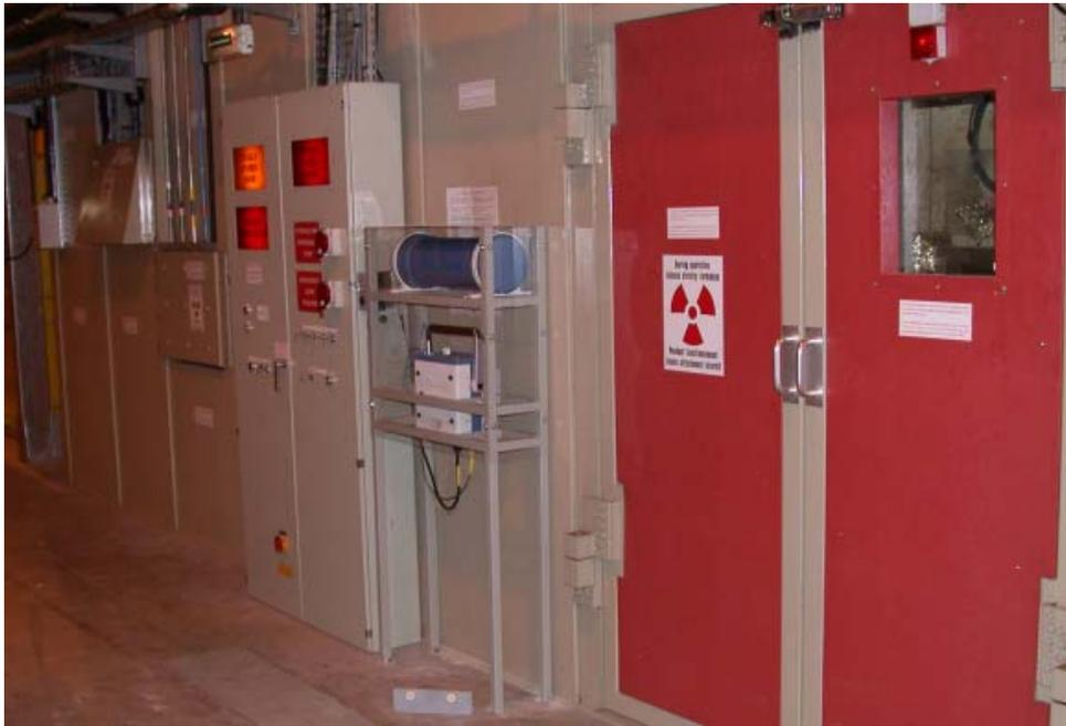
Figure 10: Picture of one of the radiation monitors installed outside an optics hutch.
